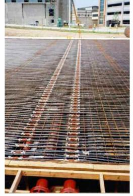
Rapid Ice is a high performance piping system for ice making with a refrigerated concrete multipurpose rink floor. Our experienced team uses the most sophisticated and reliable equipment that provides the most level and consistent concrete flatwork.
