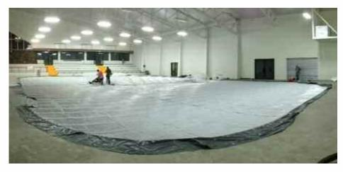
Perma Ice is pre-fabricated in 4' wide rolls, making installation fast and easy. Each roll consists of 32 heat transfer tubes spaced every 1-1/2". Because of the size and location of the Perma Ice heat transfer tubes, the floor can be fed with an "in-floor, mid-rink header," or an end-feed header, enabling 200' long mats. A single end-feed header placement cannot be done with other factory fabricated mat-type systems. End feed headers provide semi-portability.
