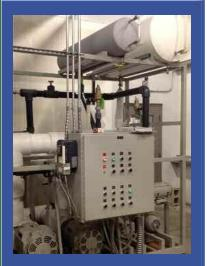
PumpStat reduces secondary pump horsepower up to 95%. It is not uncommon for a rink utilizing PumpStat to operate with only a 2 HP or 5 HP pump. This creates significant savings versus competitive systems that use large 30 HP and 40 HP pumps.
